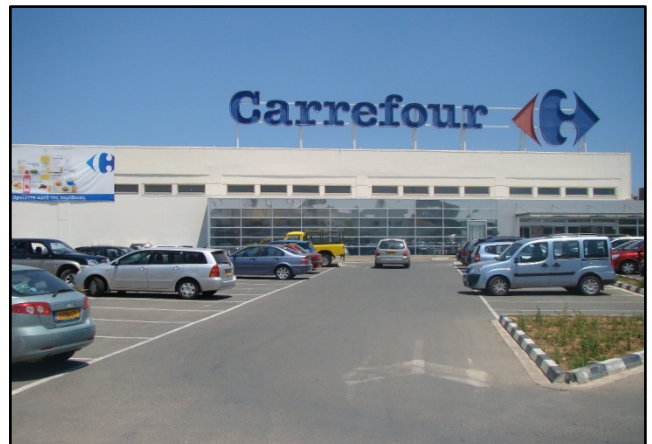
CARREFOUR PARALIMNI STORE: POWERSTAR WAS INSTALLED IN AUG 2011
