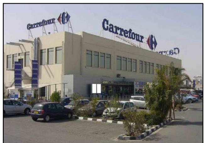
CARREFOUR COLUMBIA STORE: POWERSTAR WAS INSTALLED IN FEB 2011
