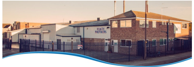
The purpose built factory based in Hull
