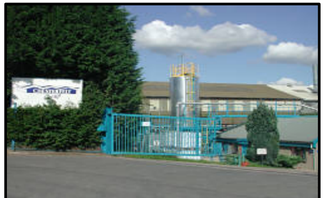
SIGNIFICANT SAVINGS: The Powerstar installation reduced annual electricity bills by around £10,000 per year
