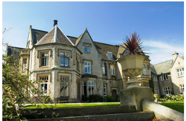
KENWOOD HALL, SHEFFIELD: located close to Sheffield City Centre
